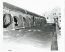
Mining Exchange_Roof_2_1976 Source: Private collection
