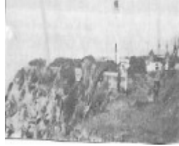
The Leading Light, Obelisk and original lower Light Keeper's quarters c.1882
