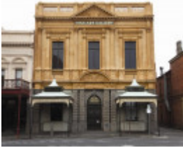
BALLARAT ART GALLERY_Restored Facade_Compressed.jpg 2010
