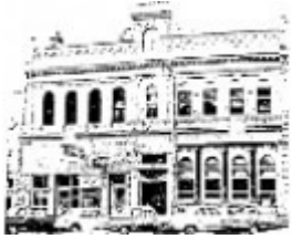
Booths Buildings - Film 1 / Frame 36 - Ballarat Conservation Study, 1978
