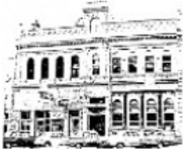
Booths Buildings - Film 1 / Frame 36 - Ballarat Conservation Study, 1978
