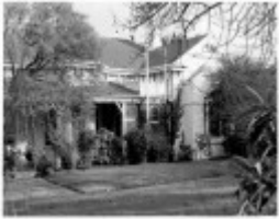
1-3 Lirrewa Grove, Caulfield South
