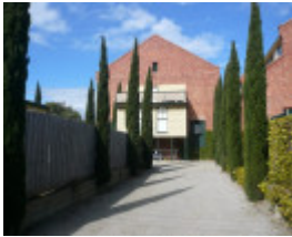
Former Vue Grand Hotel Ballroom, 13 Hobson Street, Queenscliff
