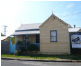
Captain Bowers Cottage, 1 St Andrews Street, Queenscliff
