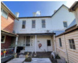
back of Kardinia house from courtyard with both extensions visible. 2023.
