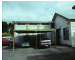
kardinia house riverview terrace belmont additions
