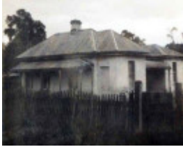
B3785 Fmr Sub Treasury Building Front View
