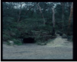
FOURTH HILL TUNNEL
