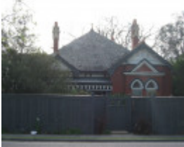
283-285 Upper Heidelberg Road
