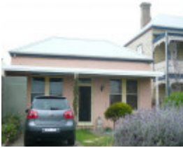
49 Mercer Street, Queenscliff
