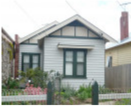
50 Mercer Street, Queenscliff
