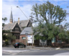
WILLIAMSTOWN PRIMARY SCHOOL NO. 1183 SOHE 2008
