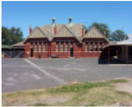
h01639 primary school no 1183 cnr cecil and parker street williamstown side view she project 2004
