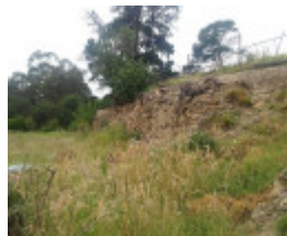
Site Visit M.Miller 21/11/13 after first day of initial investigation
