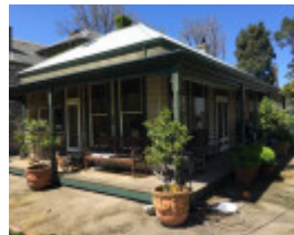
Northwest corner of mid-1980s single-storey addition.
