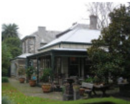
View from northwest corner of site, looking east at mid-1980s single-storey addition.
