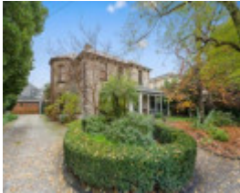
Former Presbyterian Manse from the east (Lyons Street) side. The 1991 garage building is visible at the end of the driveway on the left.
