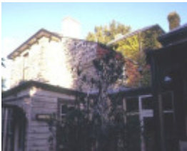
h00229 former presbyterian manse lyons st williamstown front of house she project 2003
