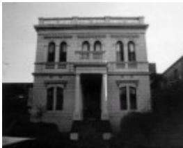
1 anne caudle centre front view superintendents building
