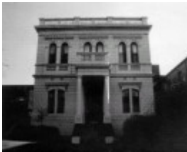
1 anne caudle centre front view superintendents building
