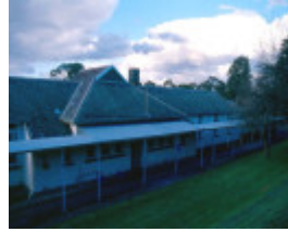
Kew Cottages Building 9 July 2004
