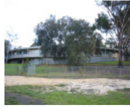
h02073 kew cottages perkin building july2004 mz
