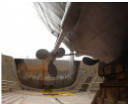
ALFRED GRAVING DOCK SOHE 2008
