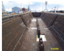
h00697 1 alfred graving dock williamstown dockyard williamstown wide view she project 2004
