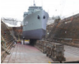
ALFRED GRAVING DOCK SOHE 2008
