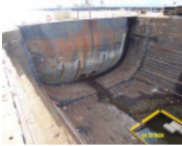
h00697 alfred graving dock williamstown dockyard williamstown close up she project
