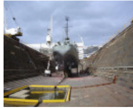
ALFRED GRAVING DOCK SOHE 2008
