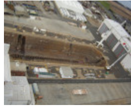
ALFRED GRAVING DOCK SOHE 2008
