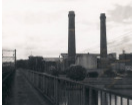
B3489 Brick Chimney Richmond Power Station
