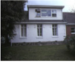
St Giles Church Gheringhap Street Geelong Former School Masters Residence Jul 1985
