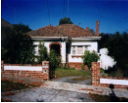
Typical English Domestic Revival villa, 9 Robina Road
