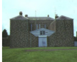
barwon park inverleigh rd winchelsea rear view homestead
