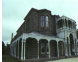
1 barwon park inverleigh rd winchelsea front view homestead
