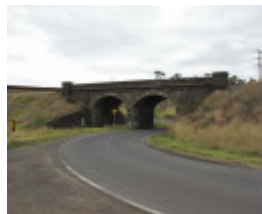
123526_Cowies Creek Rail Bridge No1_Geelong_HV_5 Feb 2010_032_resize.jpg
