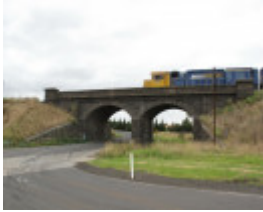
123526_Cowies Creek Rail Bridge No1_Geelong_HV_5 Feb 2010_004_resize.jpg
