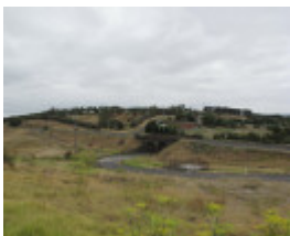
123526_Cowies Creek Rail Bridge No1_Geelong_HV_5 Feb 2010_037_resize.jpg
