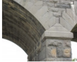
123526_Cowies Creek Rail Bridge No1_Geelong_HV_5 Feb 2010_011_resize.jpg
