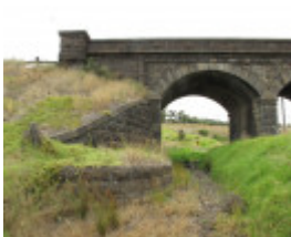
123526_Cowies Creek Rail Bridge No1_Geelong_HV_5 Feb 2010_021_resize.jpg
