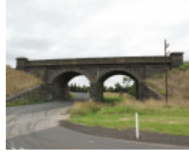
123526_Cowies Creek Rail Bridge No1_Geelong_HV_5 Feb 2010_003_resize.jpg
