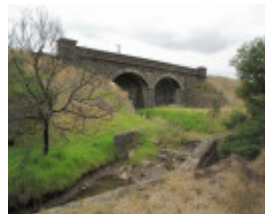
123526_Cowies Creek Rail Bridge No1_Geelong_HV_5 Feb 2010_014_resize.jpg
