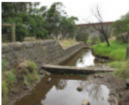
123526_Cowies Creek Rail Bridge No1_Geelong_HV_5 Feb 2010_013_resize.jpg
