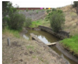
123526_Cowies Creek Rail Bridge No1_Geelong_HV_5 Feb 2010_015_resize.jpg
