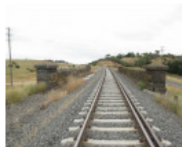
123526_Cowies Creek Rail Bridge No1_Geelong_HV_5 Feb 2010_028_resize.jpg
