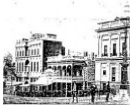
Former unicorn hotel - This view by Nettleton, taken in the 1870's shows the Hotel in its full elegance, complete with its crowning unicorn. (photograph: Nettleton's victorian Views Album, La Trobe Library) - Ballarat Conservation Study, 1978
