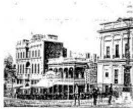
Former unicorn hotel - This view by Nettleton, taken in the 1870's shows the Hotel in its full elegance, complete with its crowning unicorn. (photograph: Nettleton's victorian Views Album, La Trobe Library) - Ballarat Conservation Study, 1978
