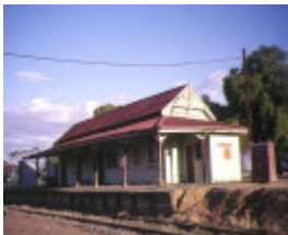
1 wycheproof railway station compelx peel street windsor track view may1984
