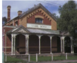
1 wycheproof court house front elevation sep1984
