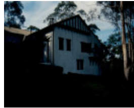
H02004 macgeorge house ivanhoe west side 02
