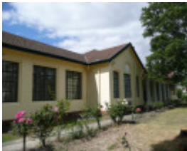
KYNETON SECONDARY COLLEGE (FORMER HIGH SCHOOL) SOHE 2008
