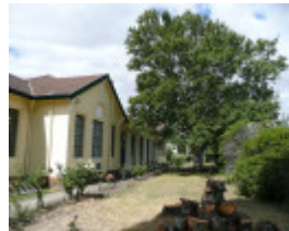
KYNETON SECONDARY COLLEGE (FORMER HIGH SCHOOL) SOHE 2008
