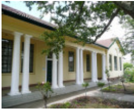
KYNETON SECONDARY COLLEGE (FORMER HIGH SCHOOL) SOHE 2008
