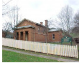
h01490 1 yackandandah court house pm1 jun03
