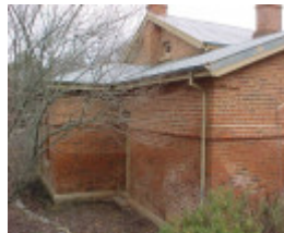
h01490 yackandandah court house 4 pm1 jun03
