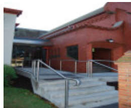
124816 Presbyterian Church Malvern new entrance 2010
