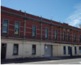
HO106 - Former Mechanics Institute, 215-217 Nicholson Street, Footscray.JPG
