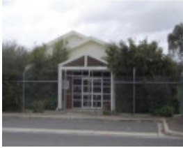
HO189(1) - Former Tottenham Bulk Stores, Beachley Street, Braybrook.JPG
