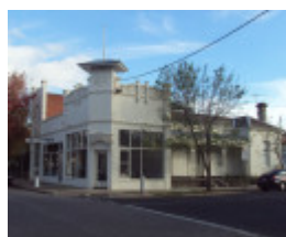
Late Edwardian shops and attached Victorian residence on the corner of Armadale Street and Fetherston Street
