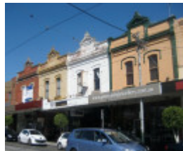
Victorian shops, 1052-1064 High Street
