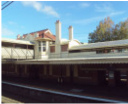
Armadale Railway Station
