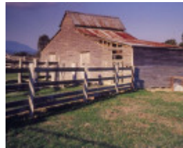
h00384 gulf station melba hwy yarraglen shearing shed west wall she project 2003
