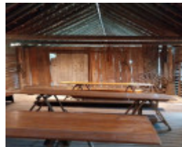
Shingle ceiling in the shed, 2023.
