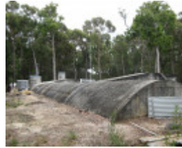
External view to the east, Feb 2008.
