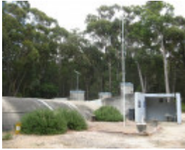
External view to the west, Feb 2008.
