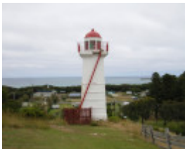
LADY BAY LIGHTHOUSE COMPLEX SOHE 2008
