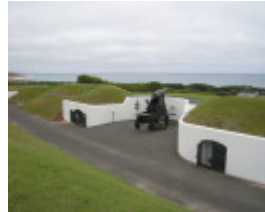
LADY BAY LIGHTHOUSE COMPLEX SOHE 2008
