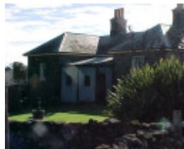
h01520 lady bay lighthouse complex cottage jun04 pm1
