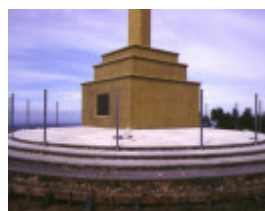
h01027 cameron memorial cross cameron drive mount macedon cross base
