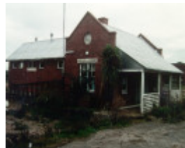
H01098 rafa barracks horse hospital demolished 1995
