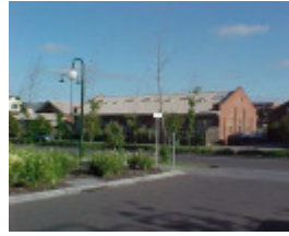
H01098 rafa barracks gun shed 2001pm1
