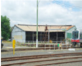
TRARALGON ENGINE SHED AND TURNTABLE SOHE 2008
