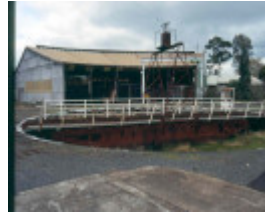
H01979 traralgon engine shed and turntable june 2001
