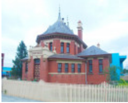
YARRAM COURT HOUSE SOHE 2008
