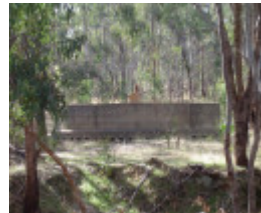
14271 Seymour Light Horse Park May 06 filtration system
