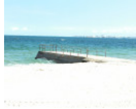
Harold St Drain Port Melbourne April 2006 002
