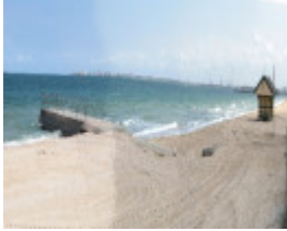
Harold St Drain Port Melbourne April 2006 001
