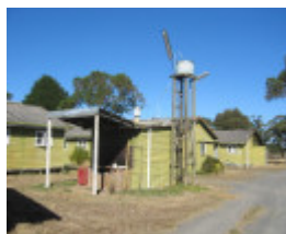
14247 Former Ballarat RAAF Base
