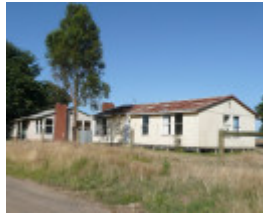
FORMER BALLARAT RAAF BASE SOHE 2008
