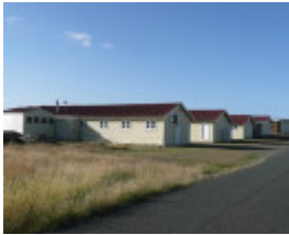
FORMER BALLARAT RAAF BASE SOHE 2008
