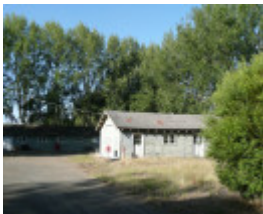
FORMER BALLARAT RAAF BASE SOHE 2008
