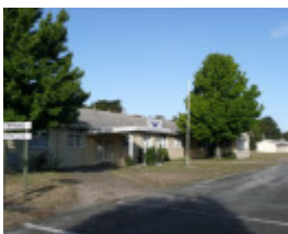
FORMER BALLARAT RAAF BASE SOHE 2008
