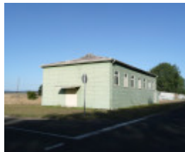
FORMER BALLARAT RAAF BASE SOHE 2008
