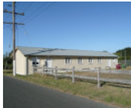
FORMER BALLARAT RAAF BASE SOHE 2008
