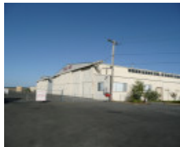
FORMER BALLARAT RAAF BASE SOHE 2008
