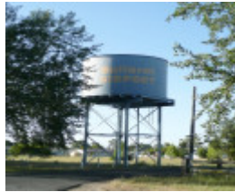
FORMER BALLARAT RAAF BASE SOHE 2008
