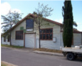
14383 Dandenong drill hall 26oct06 26
