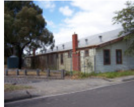
14383 Dandenong drill hall 26oct06 28
