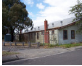
14383 Dandenong drill hall 26oct06 28
