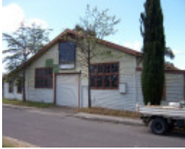
14383 Dandenong drill hall 26oct06 26
