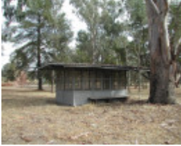
Shelter Shed, from the south east
