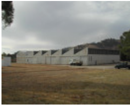
Ground Maintenance Office/Workshop
