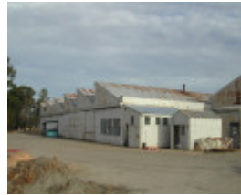
Ground Maintenance Office/Workshop
