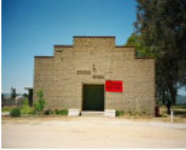
Baranduda Hall, front (west) elevation
