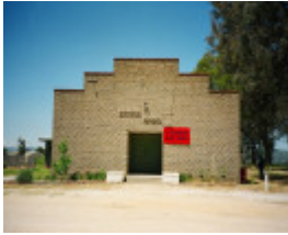
Baranduda Hall, front (west) elevation
