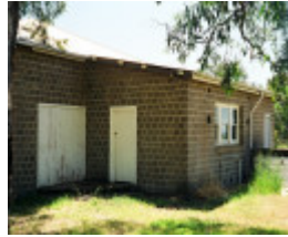
The rear of the hall, from the south east
