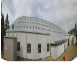
Workshop 2 from the west
