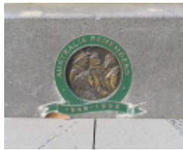
Australia Remembers plaque on the introduced concrete base of the Lorne War Memorial. Source: David Rowe, 2008.
